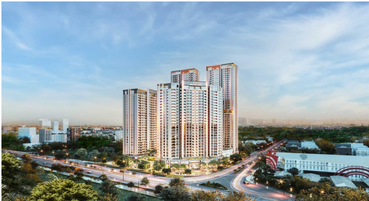
GREEN TOWER – TBS LAND
