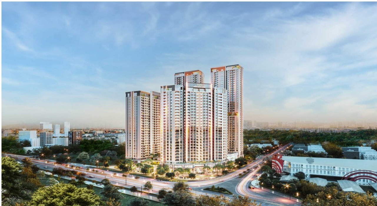
GREEN TOWER – TBS LAND
